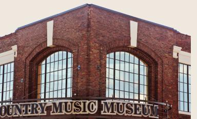
Architects Peyton Boyd and Michael Haslam of Peyton Boyd Architect PC (located in Abingdon, VA) worked with Hope's to specify the Hope's University Series solid steel windows – steel window profiles designed specifically for projects requiring historic replication of exterior putty glazed steel windows.
